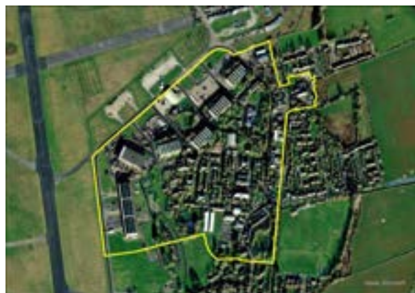
Brownfield land at Dalton Barracks
